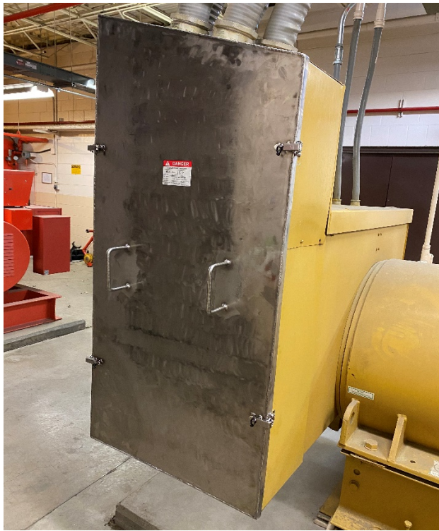
Emergency Generator Panel Door
