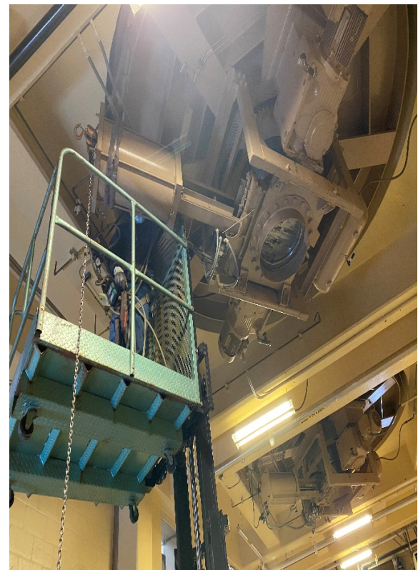
Sludge Load Out Air Cylinder Install
