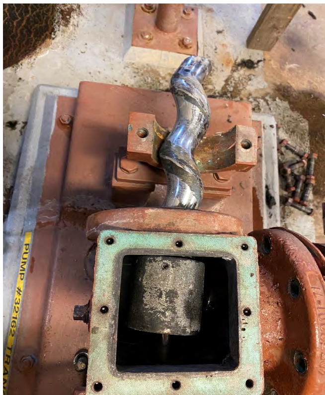
Sludge Transfer Pump Rebuild
