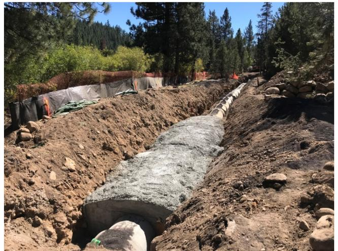
Photo 4 – Concrete Encasement Under Swale
