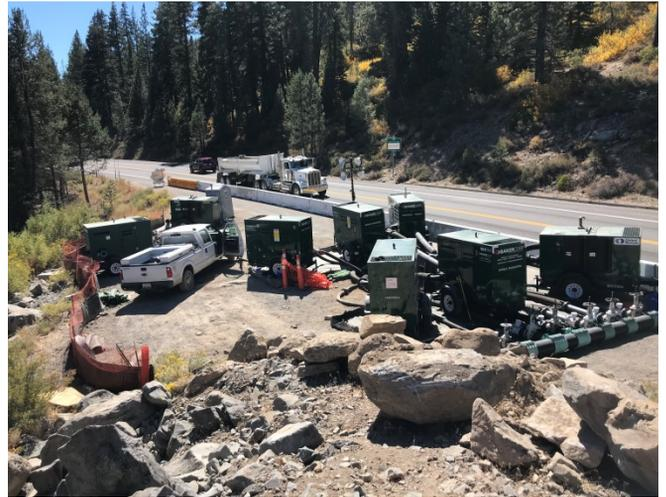
Photo 2 – Bypass Pump Station
