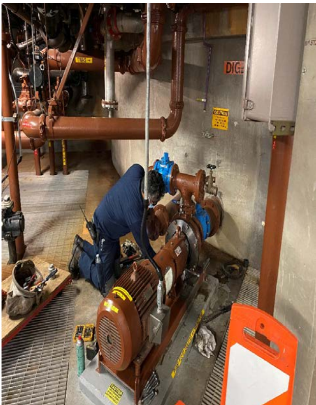
Sludge Recirculation Pump Rebuild
